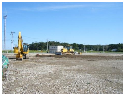
Reconstruction work in Yamamoto Town, Miyagi Prefecture
